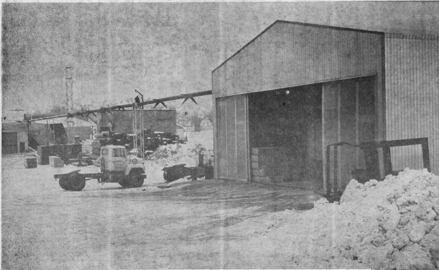
TEMPORARY SHED IN USE—His modern filter shavings shed destroyed by fire last August, Hubert Sabourin now has a temporary shavings shed in use until summer when he plans to erect a 75-foot concrete building. As seen in the picture the elevated pipe carries dust and shavings from Alexandria Moulding plant, far left, across Sandfield Street South to the temporary shed where air pollution is minimized
