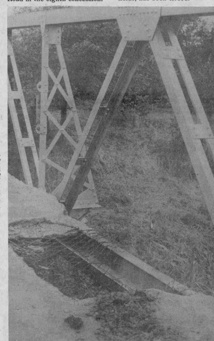
A tractor plunged through the bridge north of the seventh concession about 2 km east of the Brinston Road, leaving a hole almost 2 x 1 metres in size.
